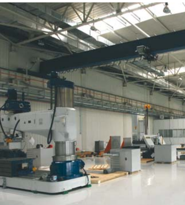
Machine component manufacturing (profile cutting, welding, base frame assembling) has been started already.
